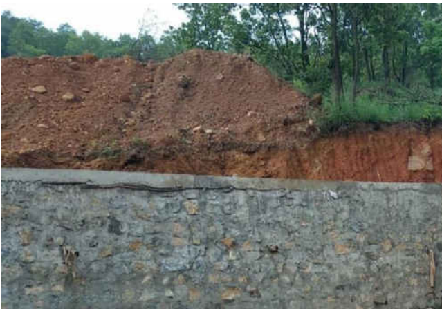
RRM wall at LILO of 132 kV MLHEP-Khliehriat Line at Mynkre
