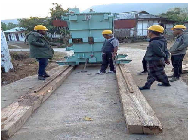
Transformer Erection Training at 33/11 kV Chukitong
