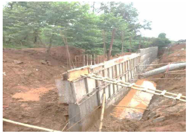
Retaining Wall at 132/33 kV Gokulnagar
