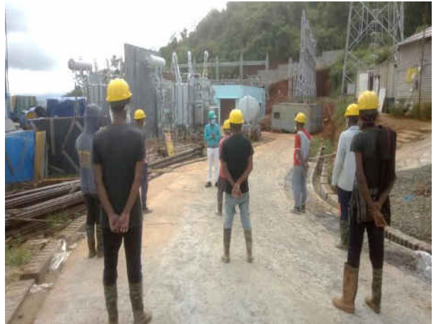
Safety Training at 220/132 KV New Shillong (GIS), Top Khongnangkong S/s
