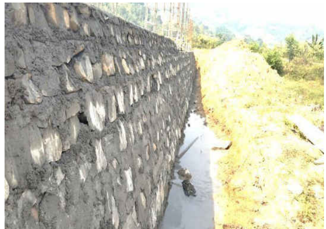
RRM Wall at 33/11kV Ando, Manipur
